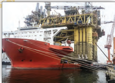
Synchronous superlift and launch
